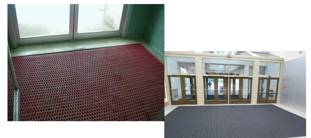
• Entry Mats – in-floor construction with drain pit
