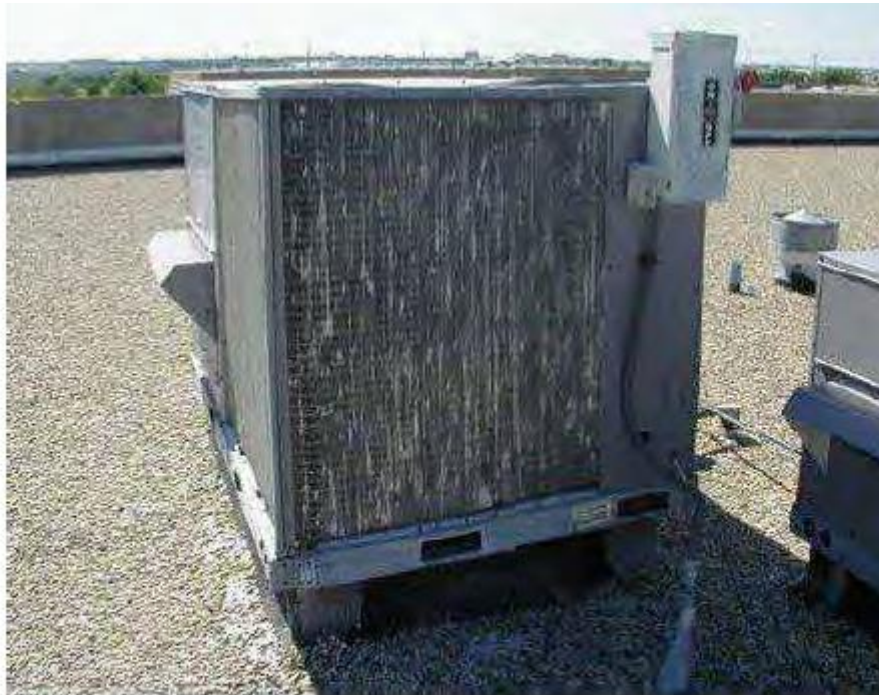
Fig. 3. Hail damaged HVAC unit
