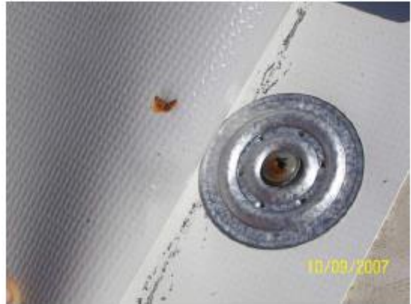
Figure 16 – View of underside of membrane at crack revealing corrosion on fastener head.
