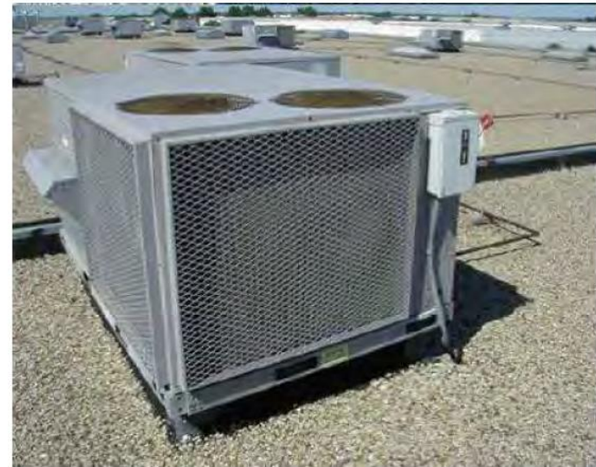
Fig. 4. HVAC unit with hail guard over cooling fins at same location as hail damaged unit in Figure 3
