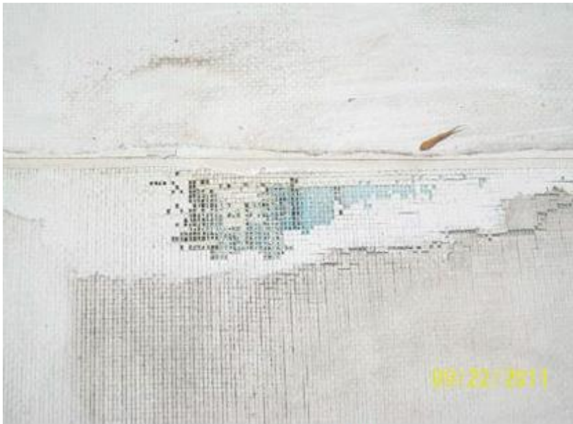
Figure 1 – Severe deterioration of TPO membrane with embrittled/loss of top coating and exposed scrim.
