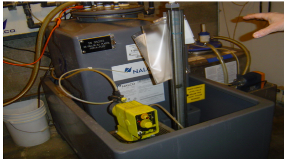
Process water tank containment
