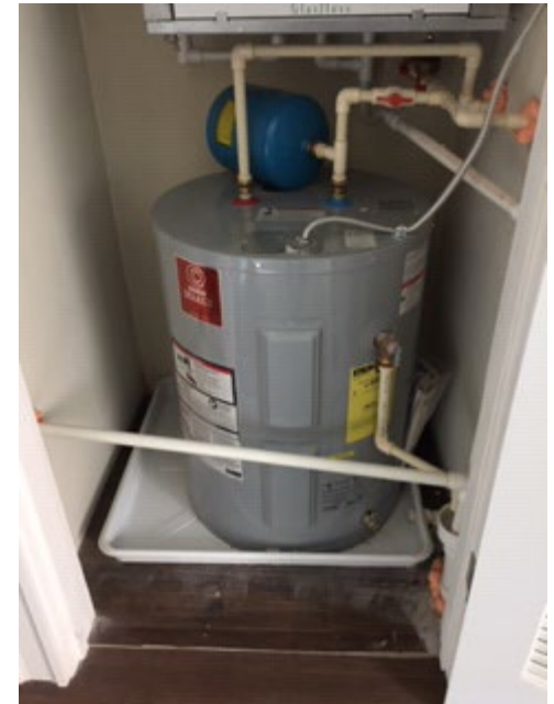
Hot water heater with drip pan and connection to drain
