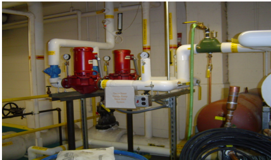
Properly posted pump shut-off instructions
