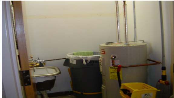
Relief valve plumbed to drain
